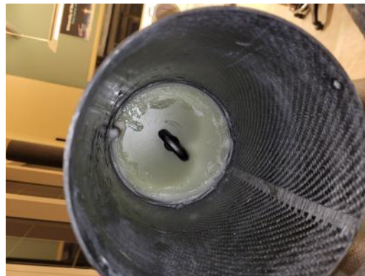
Figure 18: Constructed and Installed Fixed Bulkhead Assembly
